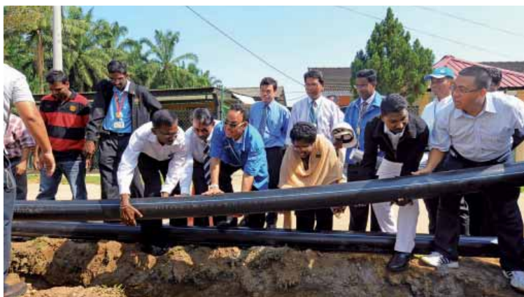
SYABAS laying water pipelines for residents at Ladang Escot, Hulu Bernam
