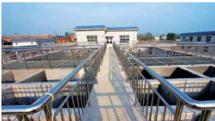
◀ Luwei Water Treatment Plant
