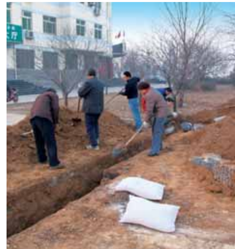
▲ Luancheng Water Project construction site
