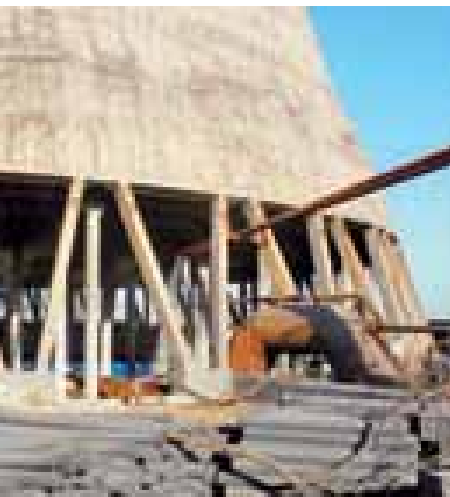
Yuanshi Industrial Water Supply Project
