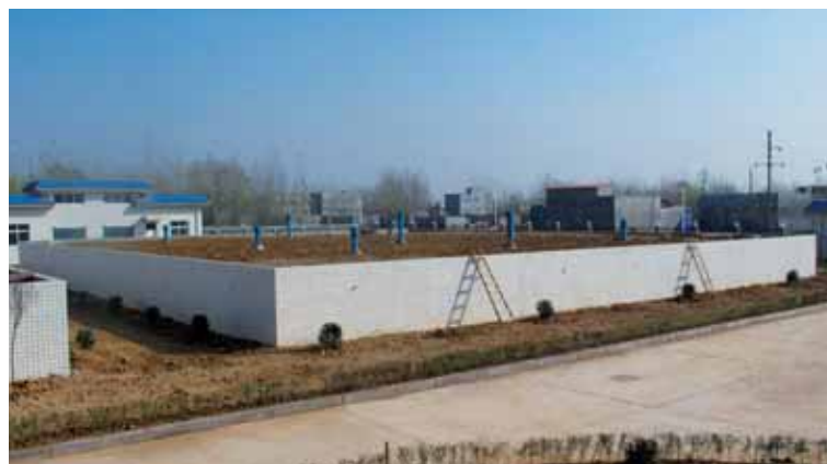
Luwei Clear Water Tank
